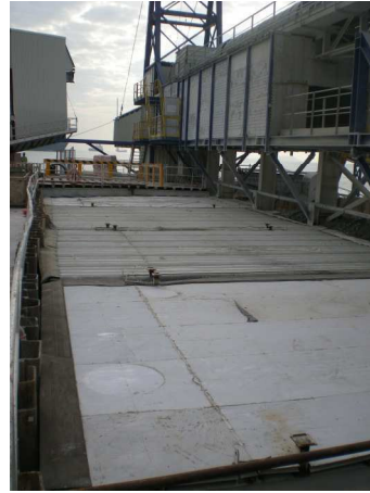
Photo 11: Noise covers at the Adit Spoil Basin
