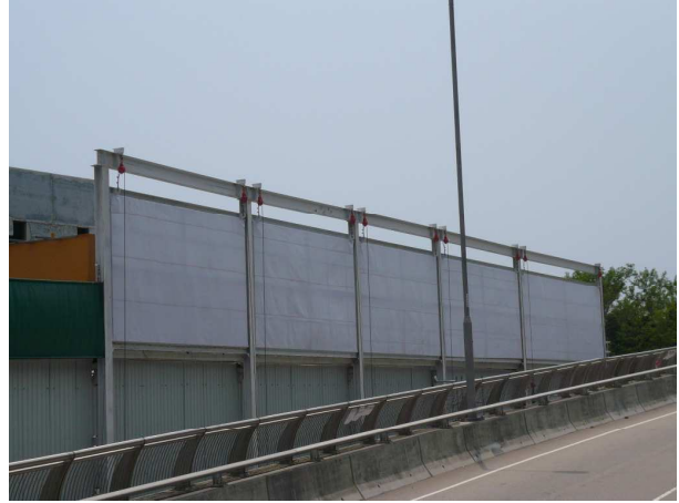
Photo 13: Noise barrier along Cyberport Road
