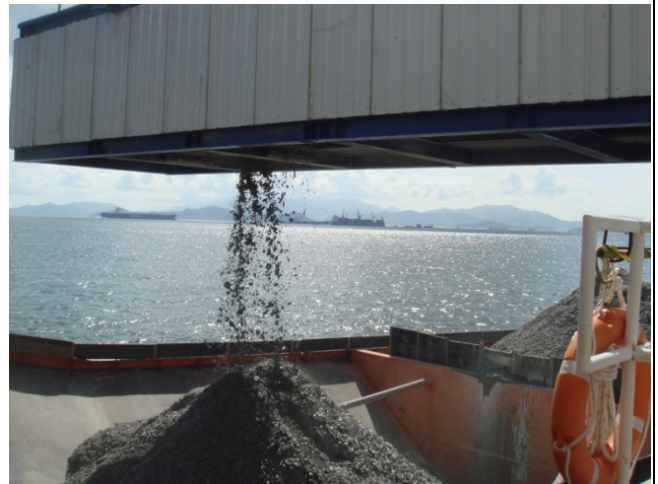
Excavated Materials Loaded Directly Onto Barges
