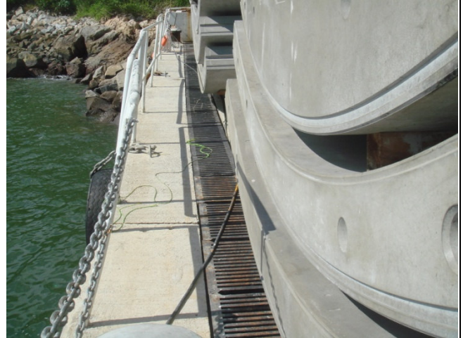
Temporary Drainage Channel
