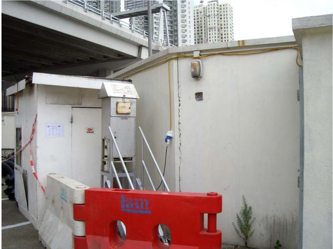
Sample photo for set-up of High Volume sampler at elevated platform
