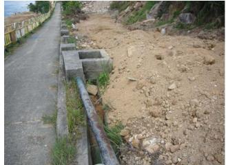
3. Soil and loose material was cumulated in the u-channel, the contractor was reminded to clean to prevent blockage of the u-channel.
