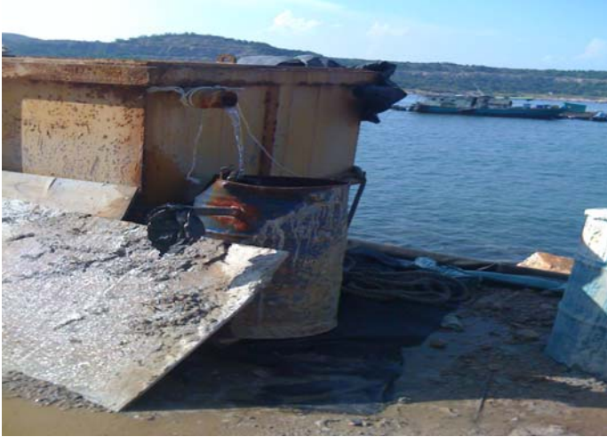
2. The de-silting facility shall be improved to avoid leakage.
