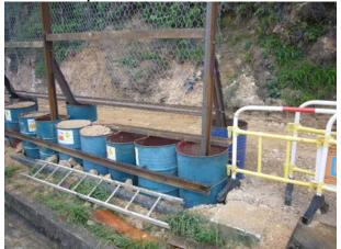
Stagnant water cumulated inside the oil drums for rock fall fencing, the contractor should provide mitigation measure to prevent mosquito breeding.
