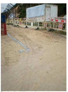
2. Dry haul road was observed, water spraying should be applied more frequently. The contractor was reminded to maintain the haul road is moist.
