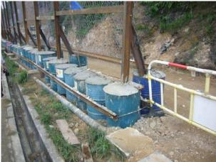
Cement was filled in the oil drums to prevent stagnant water accumulation.
