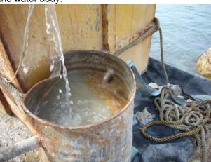
Oil firm was observed inside the sedimentation tank, the contractor was request to clean up immediately to prevent discharge to the water body.
