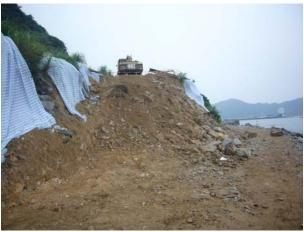
Exposed slope without protection was observed, the contractor was requested to cover the exposed surface to prevent loose material discharged into the water body from surface runoff.
