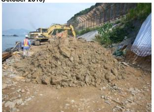
Stockpile without cover was observed near the sea side, the contractor was request to cover or remove immediately to prevent surface runoff discharged to the water body.
