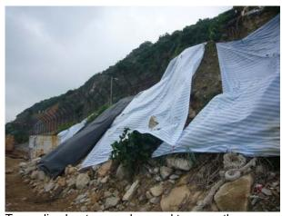
Tarpaulin sheets was observed to cover the exposed slope to prevent surface runoff.
