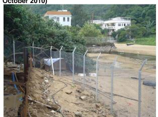
Turbidity water discharge from the sedimentation tank was observed, the contractor should improve the de-silting facility to prevent turbidity water discharged and meet the discharge licence requirement.
