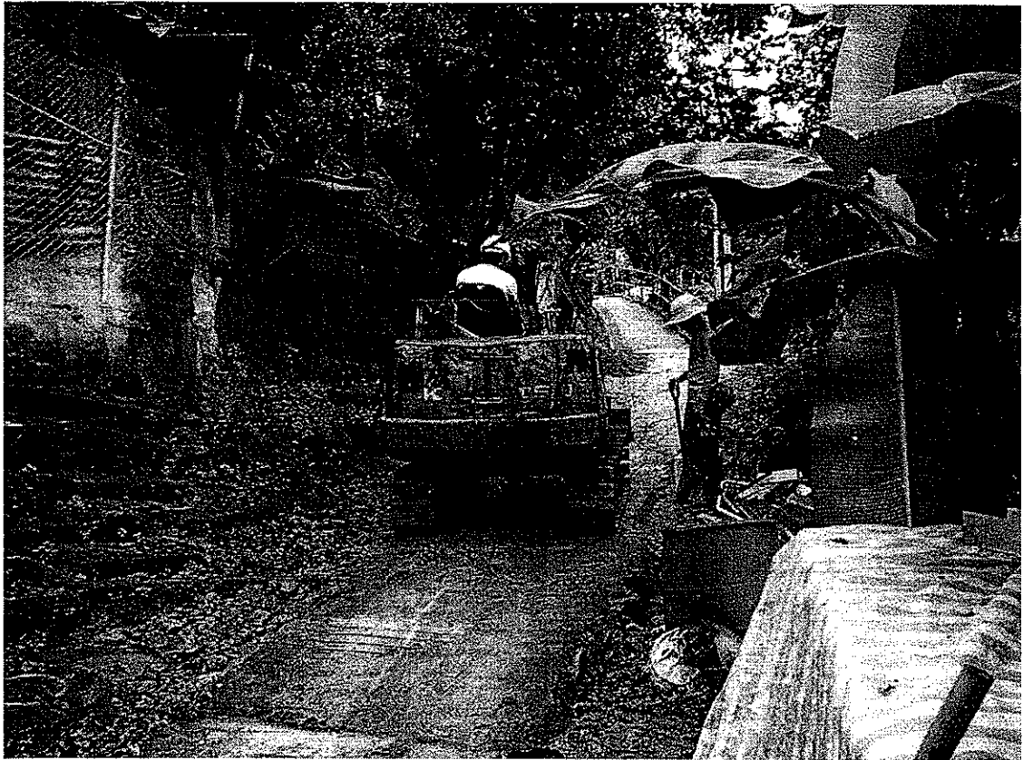
Plate 2: Pre-excavation view of alignment between MHs S51A and S50 – looking south
