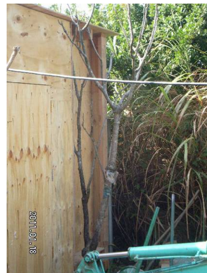
The wall was modified to avoid touching the tree branch.
