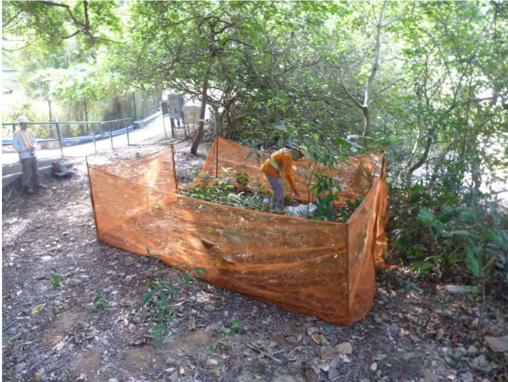
Photo 5 Overall views of the enlarged protection zone and worker placing the mulching
