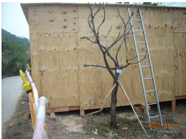
Remark 3: Protective measures should be made for the tree branch to avoid damage from the door opening.
