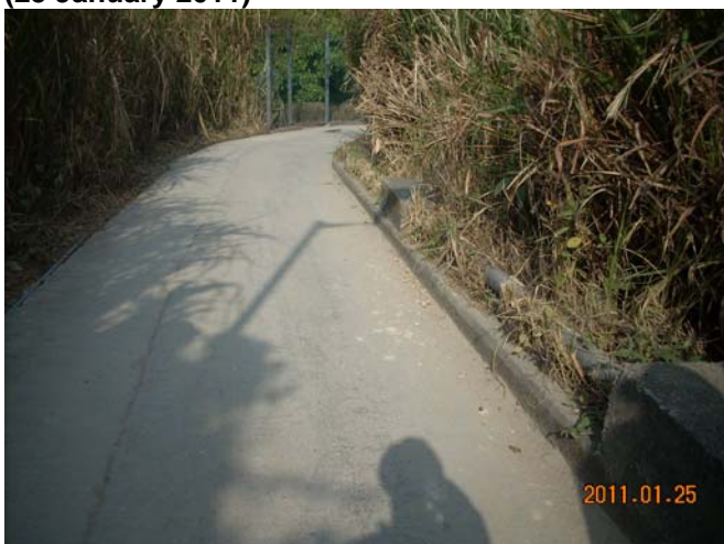
Remark 1: Dirt tails on the haul road due to transportation of construction material were observed, the Contractor should clean the road regularly to maintain site cleanliness.
