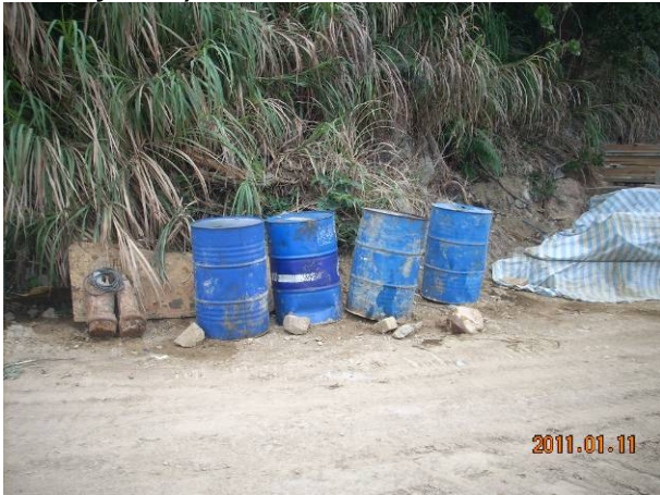
Remark 1: Free standing oil drums were observed, the Contractor should provide drip tray and covering for them.
