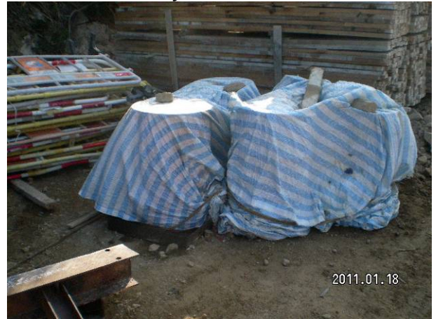
The drums were provided drip tray and covering.
