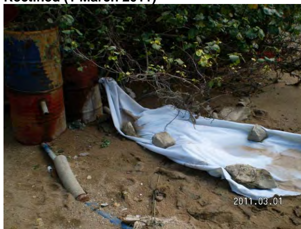
Extra filter sheet was provided at the outlet to further improve water quality.
