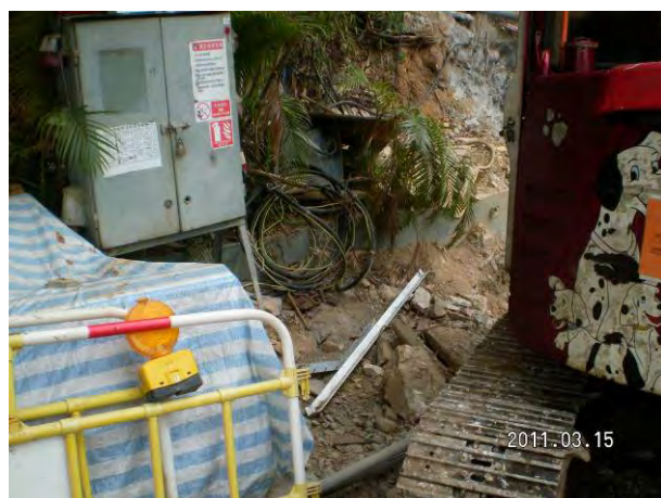
The cement bag was removed.
