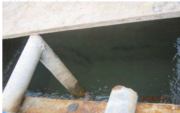
The tank was cleaned.
