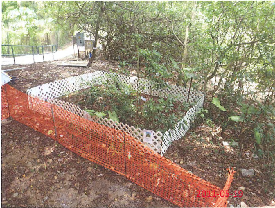
Photo 5 Overall views of the tree protection Group 1
