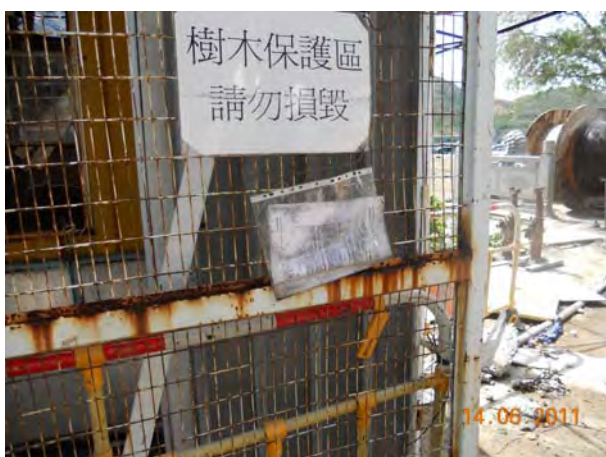
The Environmental Permit posted at the site entrances/exits was worn after rainstorm,
