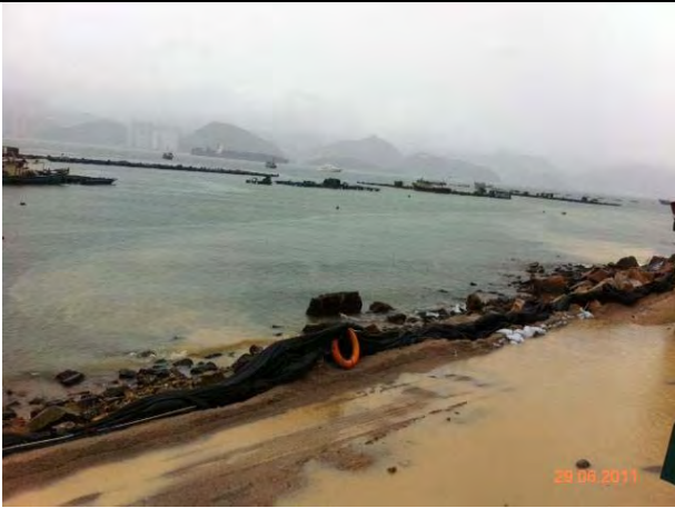
Muddy runoff to the marine body was observed after heavy rainstorm, the Contractor is reminded to improve the drainage system to avoid overflow of muddy water especially in wet season.
