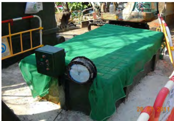
The tank has been covered. (Rectified on 27-7-2011)
