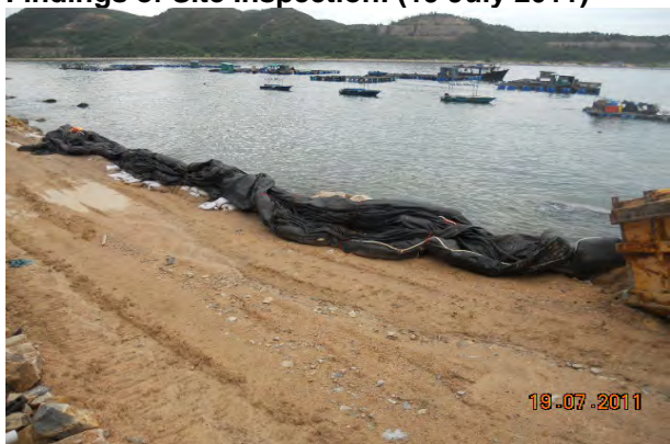
Tarpaulin sheet should be put back to sea to restore de-silting functioning.
