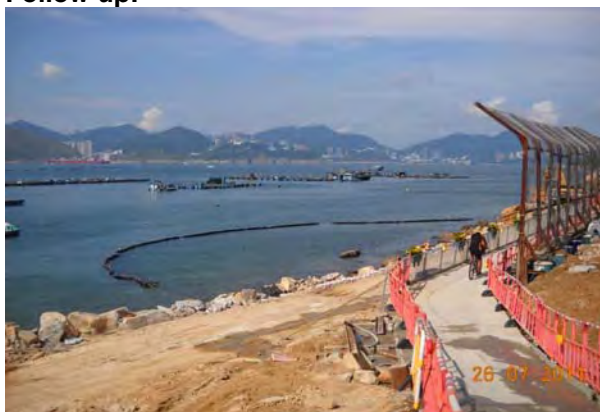
Tarpaulin sheet has been deployed into the sea. (Rectified on 27-7-2011)
