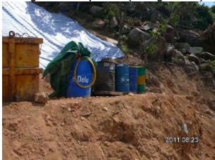
The Contractor should provide enough drip trays or covering for the chemical containers.
