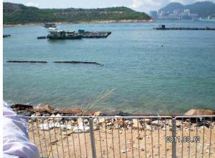
The silt curtain was not completely enclosed the sea bank. The Contractor should modify the curtain to ensure its de-silting effectiveness.
