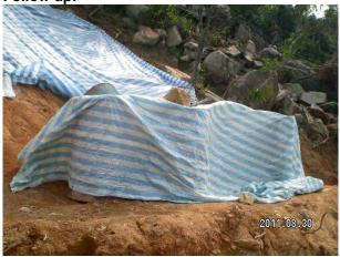
The containers were provided drip trays and covered (Rectified on 30-8-2011)
