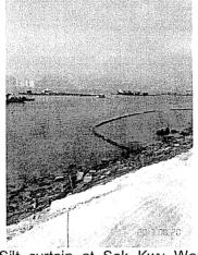
Silt curtain at Sok Kwu Wan was observed broken, the contractor was reminded to provide proper maintenance to make sure the silt curtain is functional.
