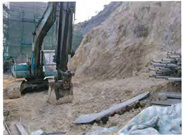
The stockpile of soil material has been backfilled.
