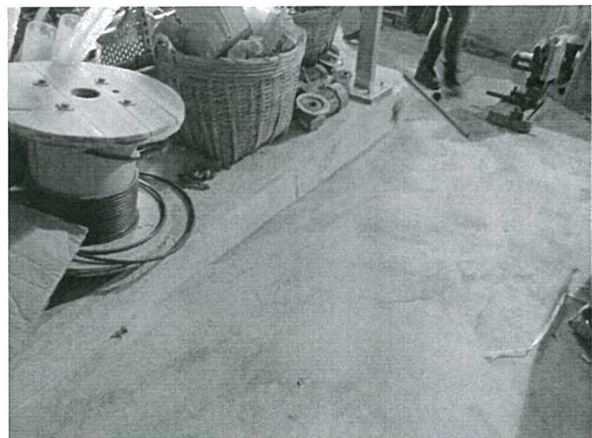
The empty cement bag has been removed.
