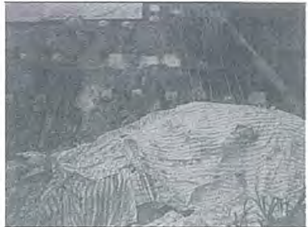
The stockpile was better covered.
