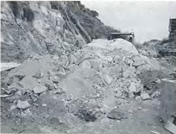
The Contractor was reminded to better cover the stockpile with impervious sheet to reduce dust generation
