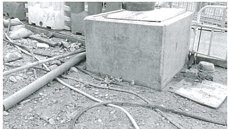
The empty cement bag was removed and good housekeeping was kept.
