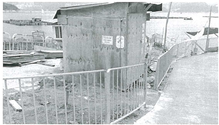
The water barriers were removed.
