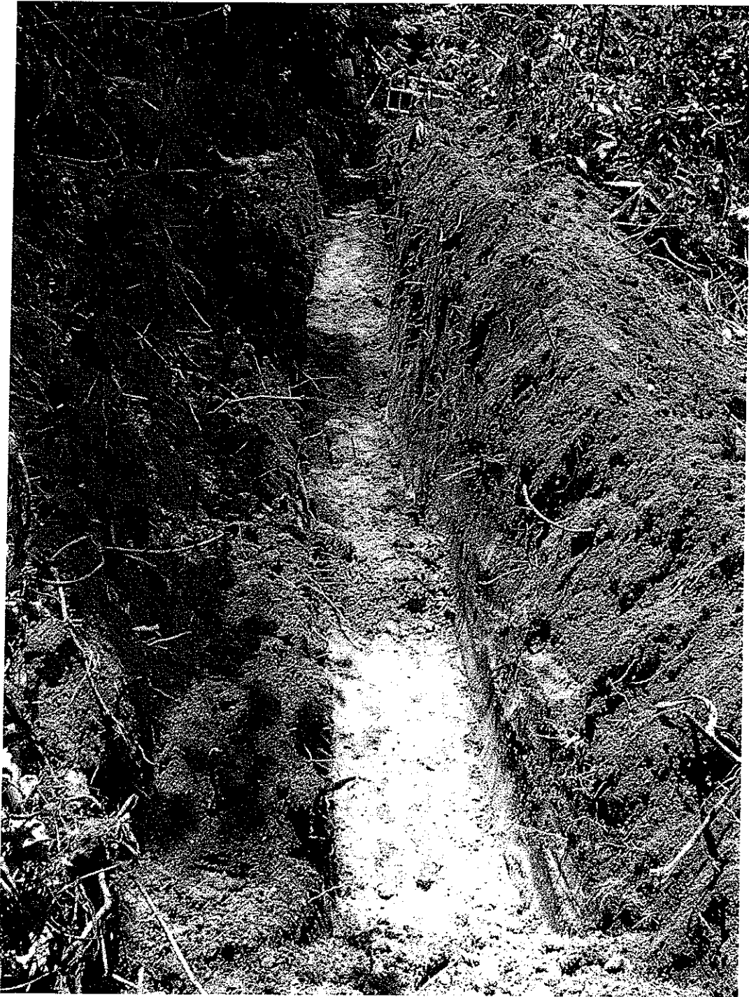
Plate 3: Post-excavation view of the alignment between MHs S54 and S52 – looking south
