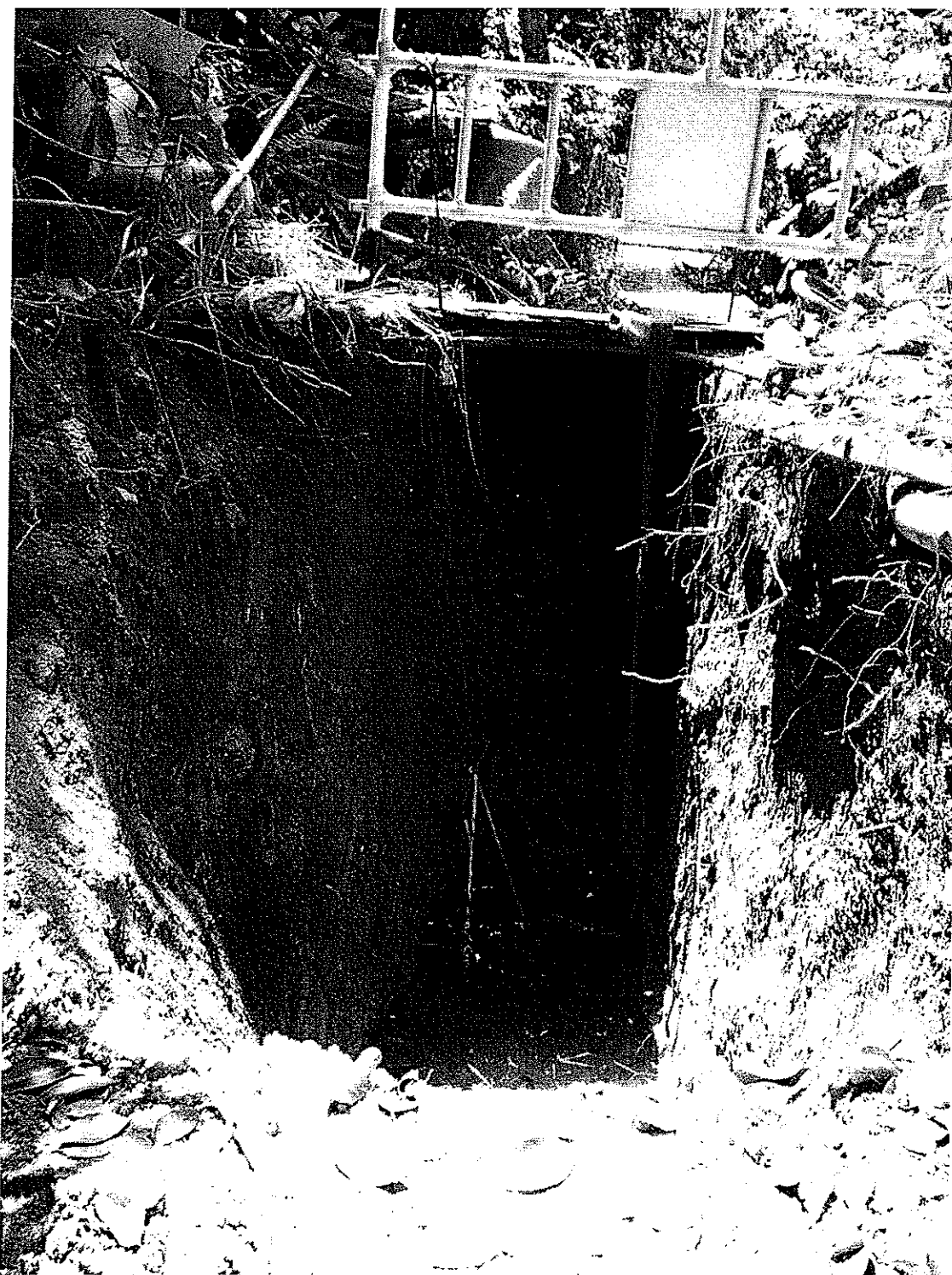
Plate 4: Deeper sondage excavated at MH S52 – looking south
