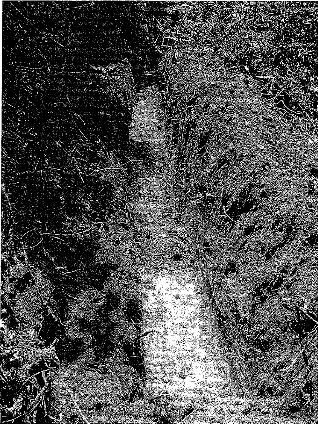
Plate 3: Post-excitation view of the alignment between MHs S54 and S52 – looking south
