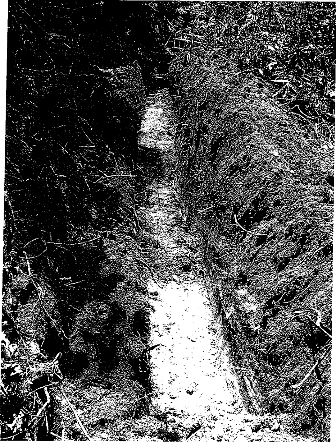
Plate 3: Post-excavation view of the alignment between MHs S54 and S52 – looking south
