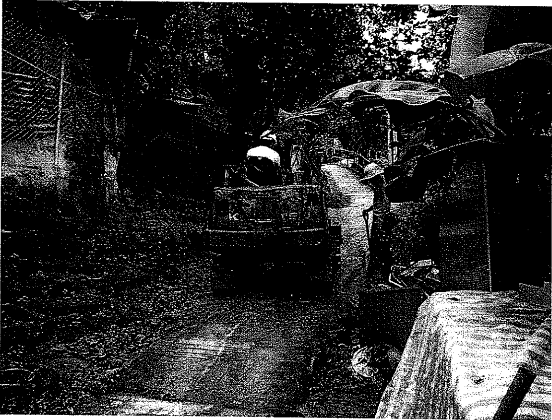
Plate 2: Pre-excitation view of alignment between MHs S51A and S50 – looking south
