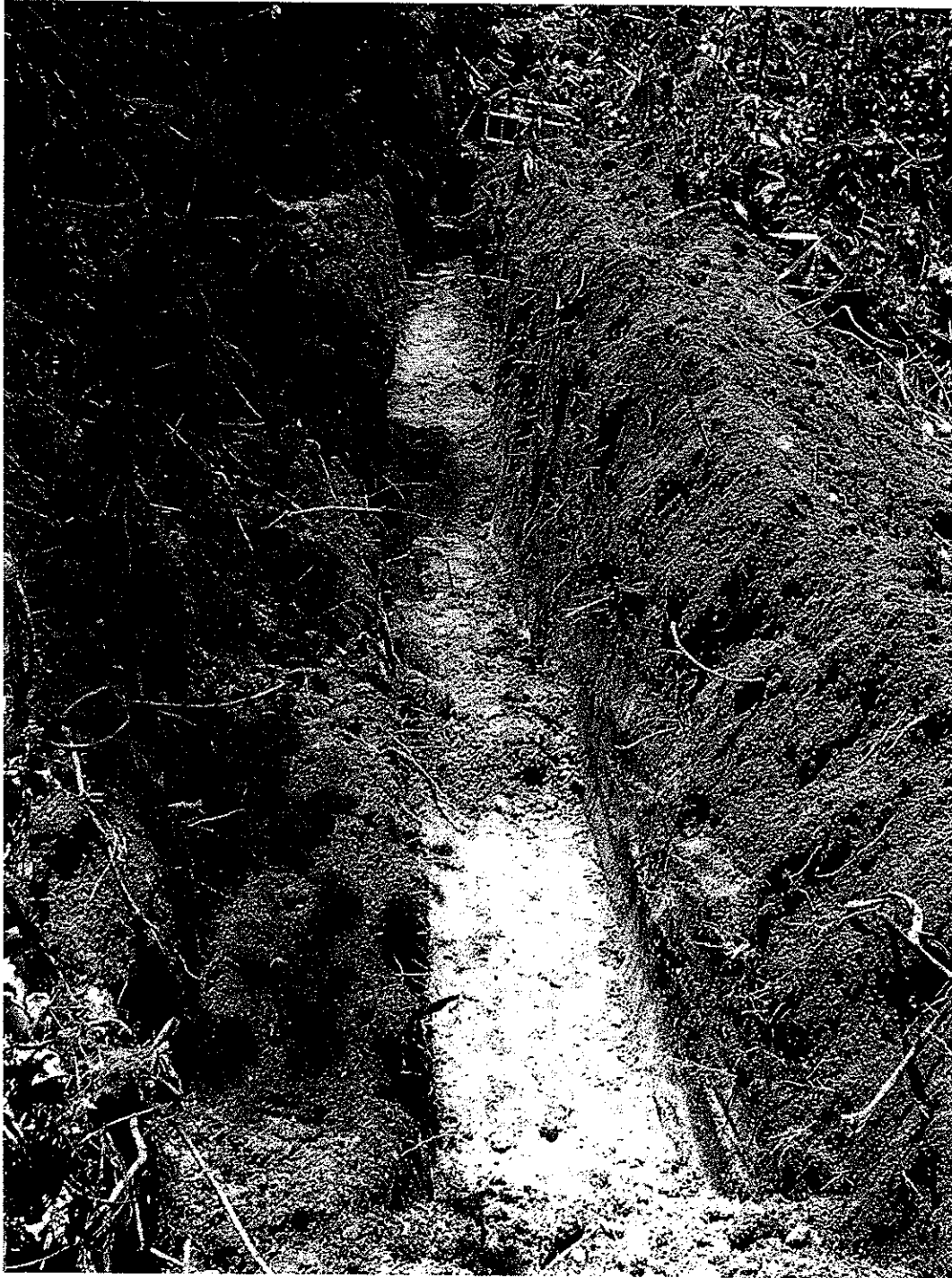
Plate 3: Post-excavation view of the alignment between MHs S54 and S52 – looking south
