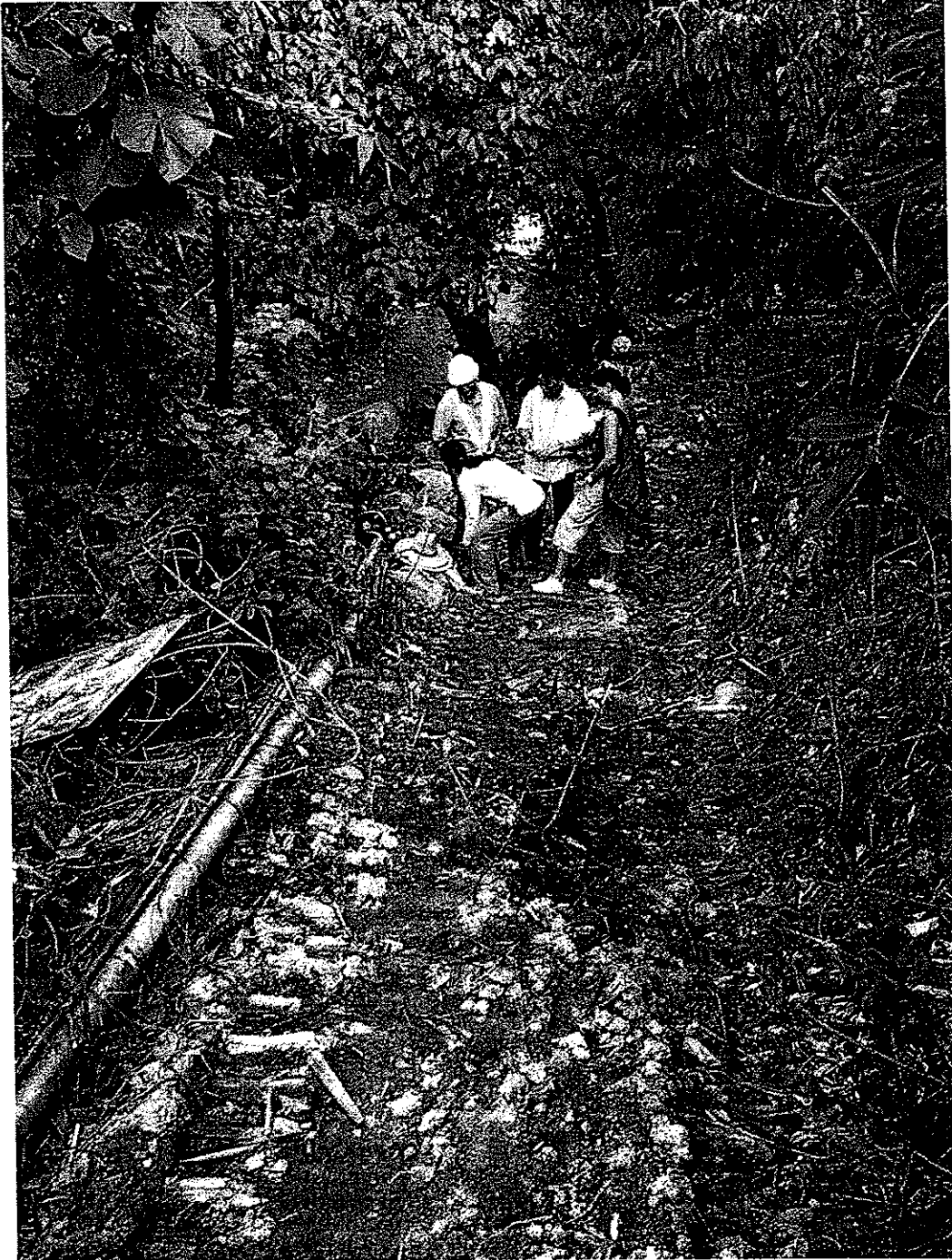
Plate I: Pre-excavation view of the alignment between MHs S52 and S54 – looking north
