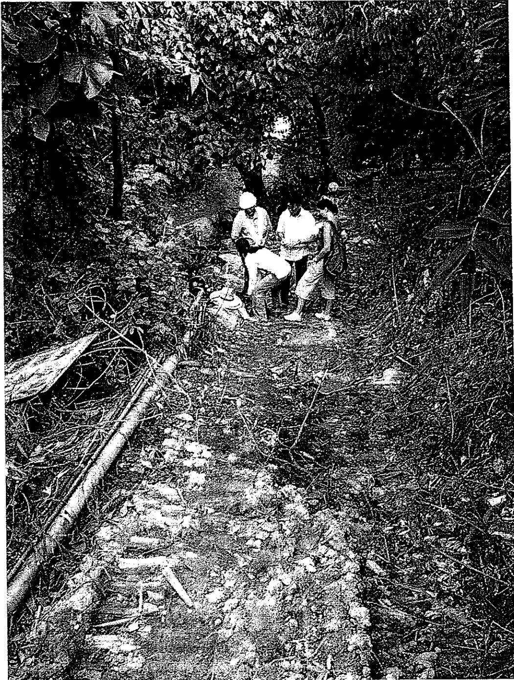
Plate 1: Pre-excitation view of the alignment between MHs S52 and S54 – looking north
