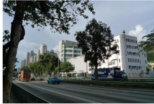
Photo C05 GIC1 Tuen Mun Church and Tuen Mun Tseng Choi Street Joint-user Complex
