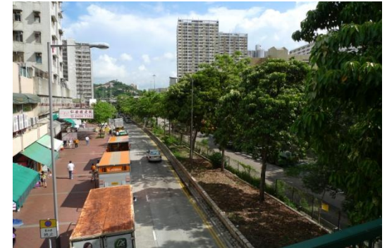
Photo A06 LR4 Street trees along Tuen Mun Road west of Chi Lok Fa Yuen and east of On Ting Estate
