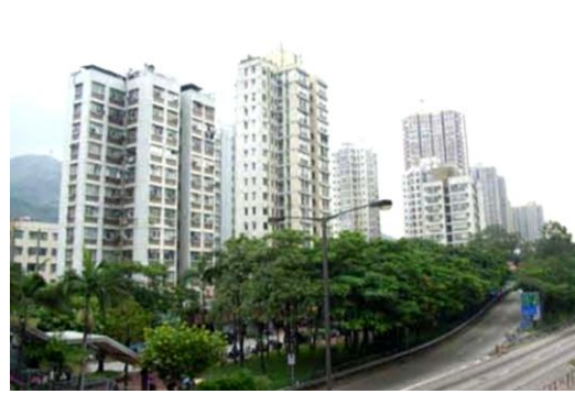
Photo C20 R3 Residential Area along Yan Oi Tong Circuit
