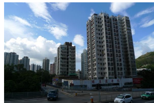
Photo C15 R2 Residential Area along Yan Oi Tong Circuit
