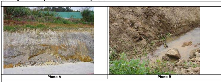
**Photo A and Photo B:** Exposed slope has hard paved in some area, However, the Contractor is reminded to enhance the water mitigation measures, such as sand bag should be erected under loose open slope.
