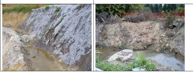
Exposed slope has been well compacted and de-silting facilities was provided in water channel to enhance the water mitigation measures.
