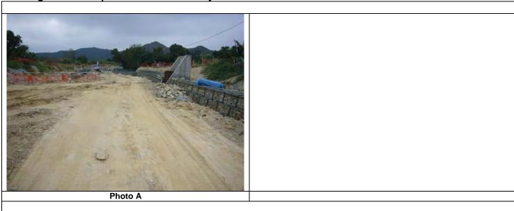
Photo A: Dry haul road was observed, the Contractor was reminded to provide water spraying more frequently.
