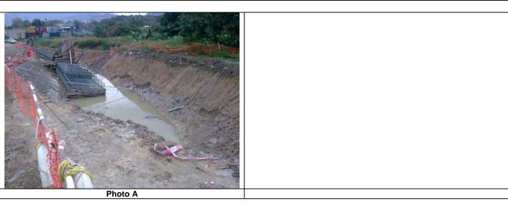
**Photo A:** The stagnant water accumulated is observed. The Contractor was reminded to drain water away or apply larvidical oil to prevent mosquitoes breeding.
