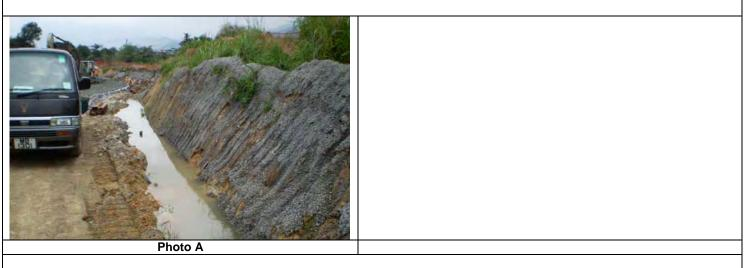
**Photo A:** Stagnant water was observed during the site inspection. Pump out the stagnant water or level off the land was reminded to be undertaken to prevent mosquitoes breeding
