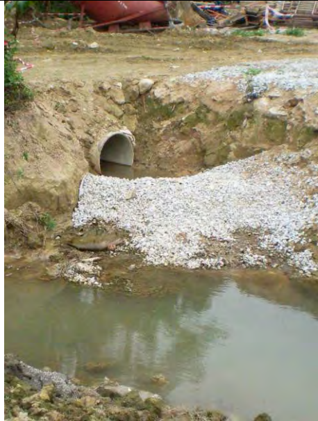
The rock barrier was repaired at channel MUP01
