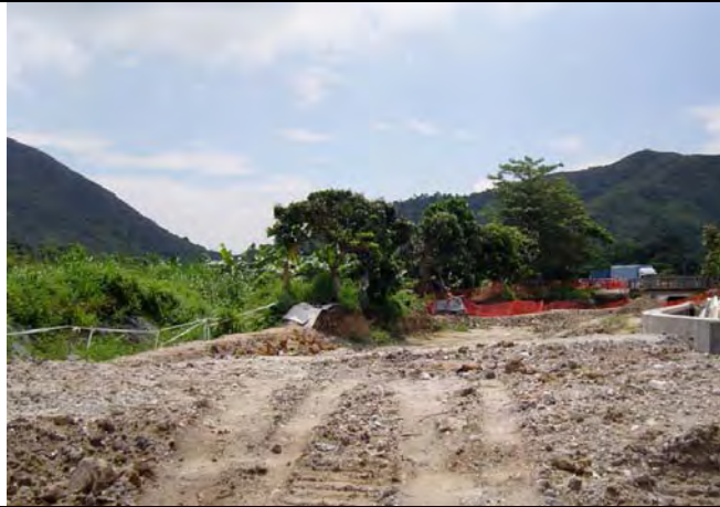
Soil stockpiled on the site was disposed off site. (TKL 07)
