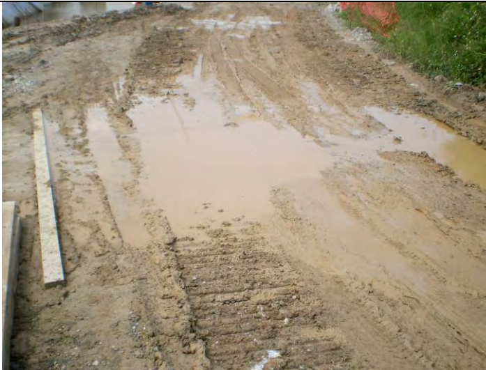
1. As a reminder, after rainfall the contractor was reminded to clear the stagnant water within the site to prevent muddy water run-off. (TKL 02 & MUP 02)
