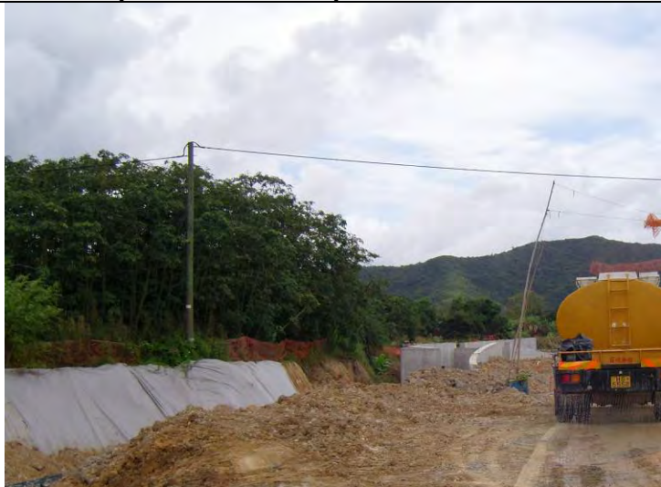
Exposed stockpile material was removed
