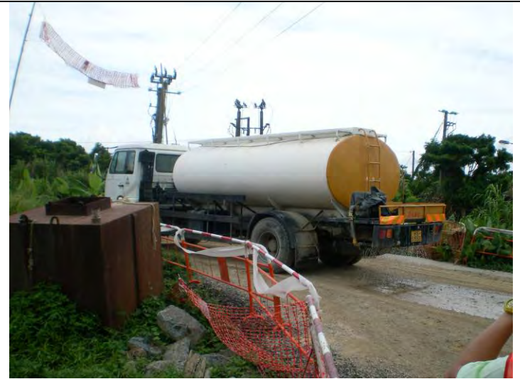
Water spraying was applied.
