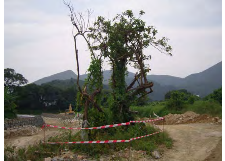
Proper protection was provided to retained trees. (MUP05)
