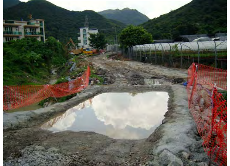
Dry wheel-washing facility was maintained in proper function. (MUP04)
