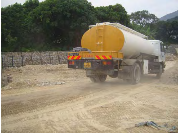
Water spraying was applied
