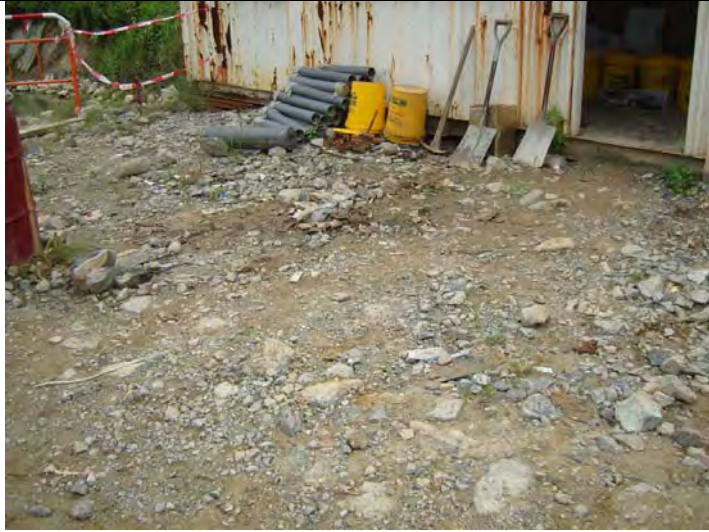
Scattered of C&D waste and general refuse were removed, (TKL02)
