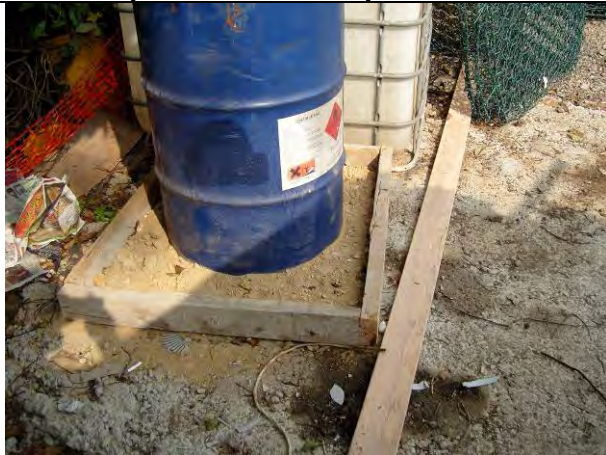
Drip tray was applied for chemical container.[TKL07]
