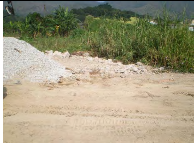
The dirt by oil leakage was cleared. [MUP05]
