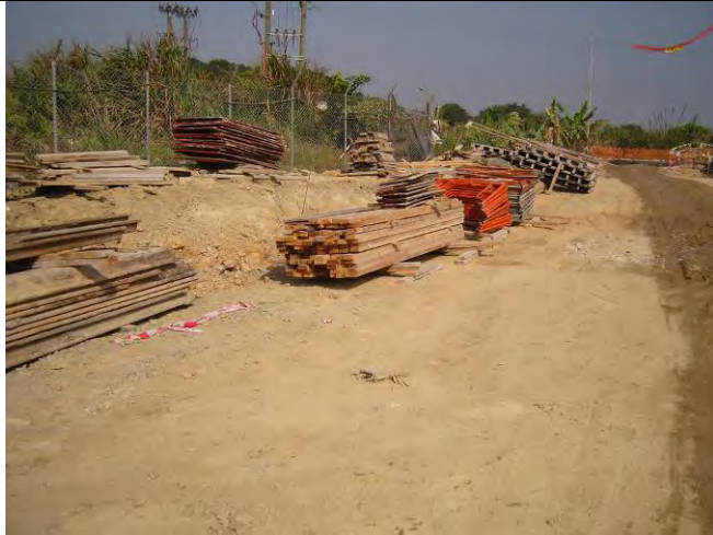
Remark 1: Dismantled plant was removed from construction site [TKL02]
