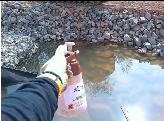
Larvicidal oil was sprayed to stagnant water for mosquito control.
