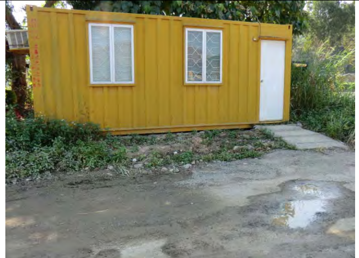
Remark 2: General refuse was cleaned up. (MUP05)
