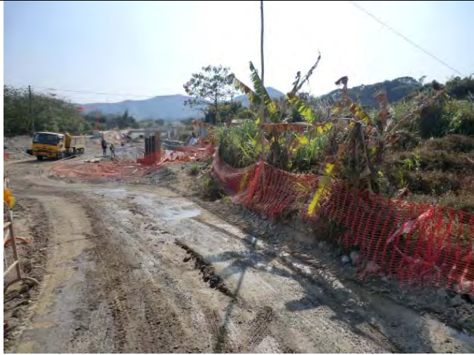
Remark1: Waste generated from construction work was removed. [TKL 02]
