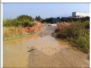
Overflow of turbid water from wheel-washing facility was observed. The Contractor was reminded to pump away turbid water for desilting before discharge and prevent further runoff.
