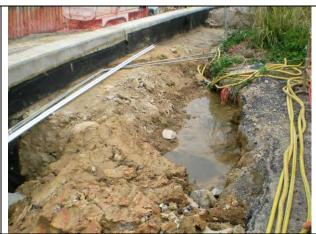
The stagnant water accumulated should be drained away or applied larvidical oil to prevent mosquitoes breeding. [TKL02]
