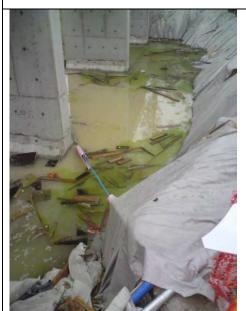
The C&D material floating on the channels should be removed immediately. Also, the Contractor was reminded to implement desilting facilities, such as set up gabion prior discharge to reduce the SS content.
