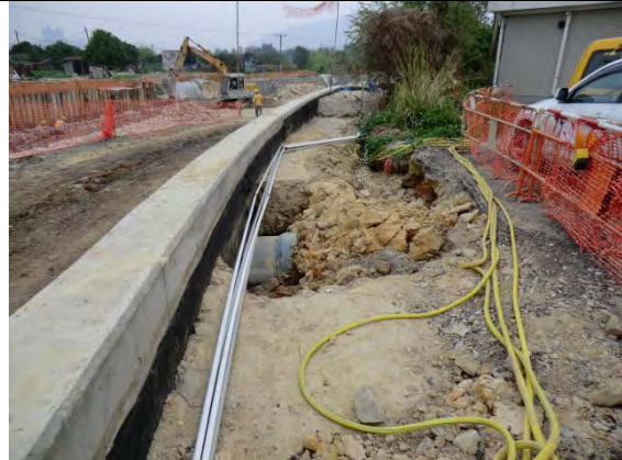
The stagnant water was eliminated to prevent mosquitoes breeding. [TKL02]
