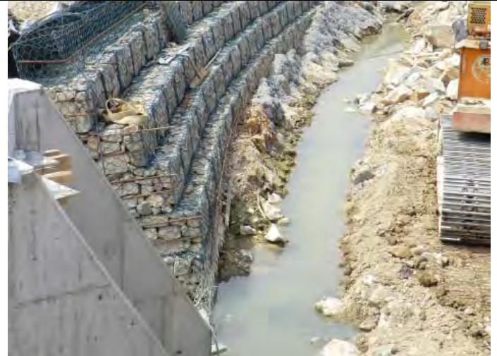
Construction materials were disposed properly.[TKL07]
