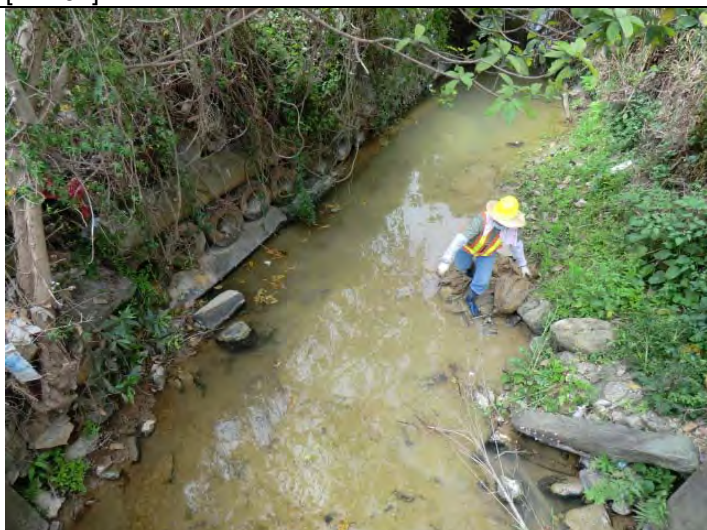
The waste in the stream was removed. [MUP05]
