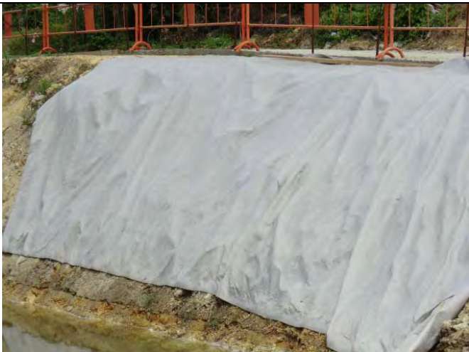
Exposed slope was covered against soil erosion (MUP04)
