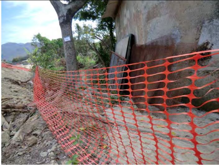
Remark 1: The safety mesh was properly maintained for tree protection measures.[TKL07]
