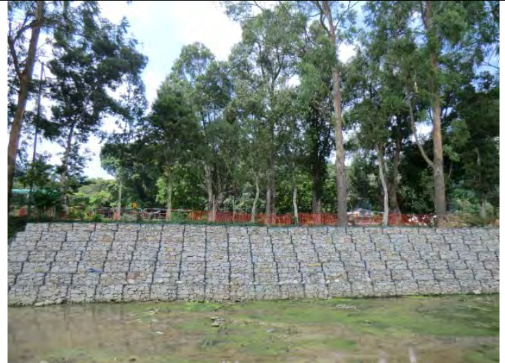
A fallen tree branch has been removed
