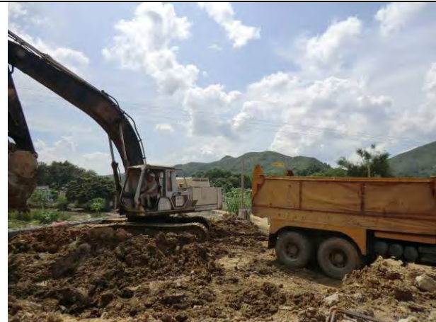
Photo 2: The stockpile was cleared.
