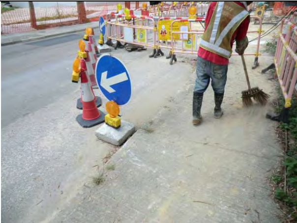
Photo 3: The mud on public access was cleaned.
