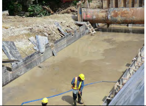
Photo 2: Floating C&D waste was removed.
