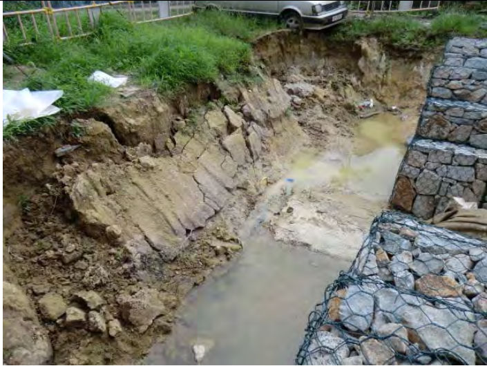
Photo 1: C&D material in the channel was removed.
