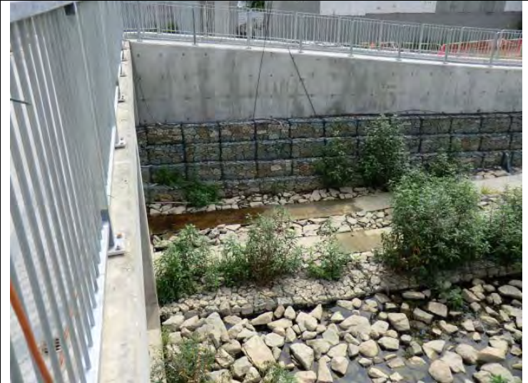
Photo 2: C&D material in the channel was removed.
