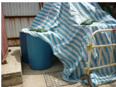
Photo 3: Chemical drums without drip tray were found in PTW
