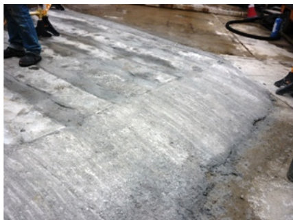
Photo 1: The piles had been paved with cement
