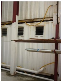
Photo 3: The water leaking from the toilet was reduced
