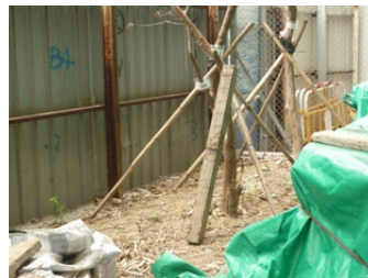
Photo 4: The accumulated materials near the site hoarding were cleared.
