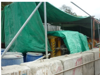
Photo 3: Chemical drums without drip tray were found in PTW
