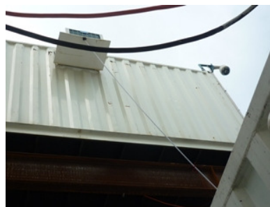
Photo 2: The temporary duct had been provided to air-conditioner
