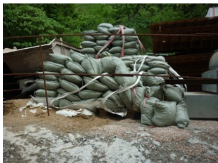
Photo 1: The leakage sand bags were found
