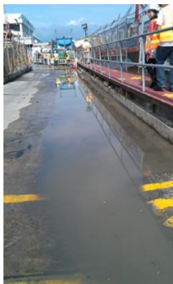
Photo 1 The accumulated water was found in access road
