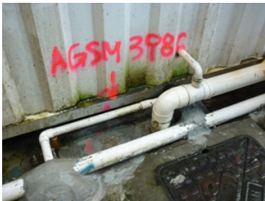
Photos 4 and 5 : Leaking pipe was found hang near container
