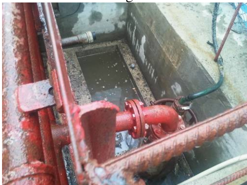
Photo 3: The rubbishes were removed in the pit near vehicles washing facilities.
