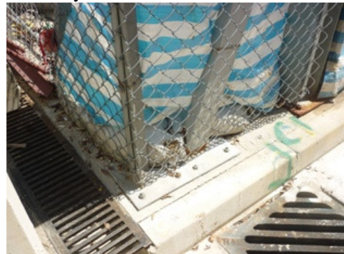
Photo 2: Some leaking sand bags were found near site boundary fences
