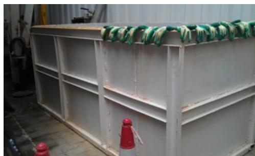
Photo 2 The accumulated water was still found in the container since last inspection
