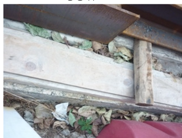
Photo 2 Accumulated leaves were found in PTW
