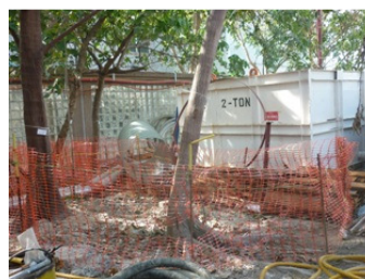
Photo 2: Tree-protecting fence was reinstalled
