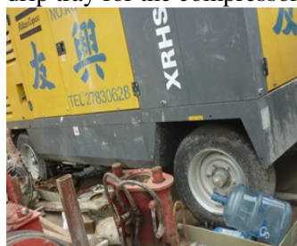
Photo 2 : Some miscellaneous articles were found in drip tray for the compressor.
