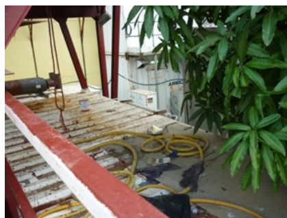
Photo 2 Unused chemical materials were found on roof of workers resting area
