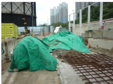
Photo 3 The cement mixer had been removed
