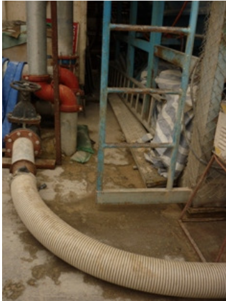
Photo 1 Mud was found underneath the treatment tank was cleared
