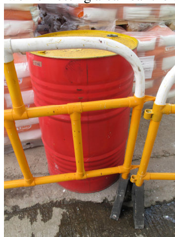
Photo 2 Chemical drum without drip tray found in worker resting area near the entrance
