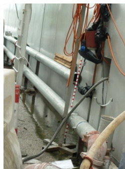
Photo 4 Chemical drum near chemical storage was found without drip tray
