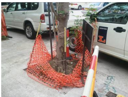
Photo 1 The protection fencing for the tree was found damage at the car park area
