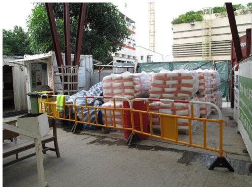
Photo 3 Stocking of chemicals in the worker resting area near the entrance shall be avoided
