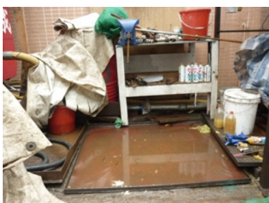
Photo 1 Water accumulation was found in drip tray near air compressor
