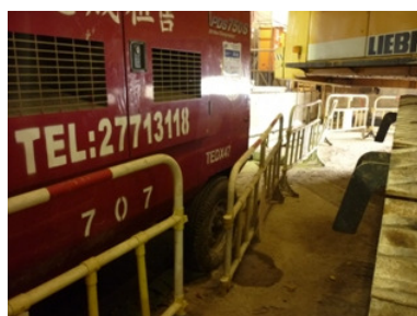
Photo 5 The pump was silted up with mud near the access
