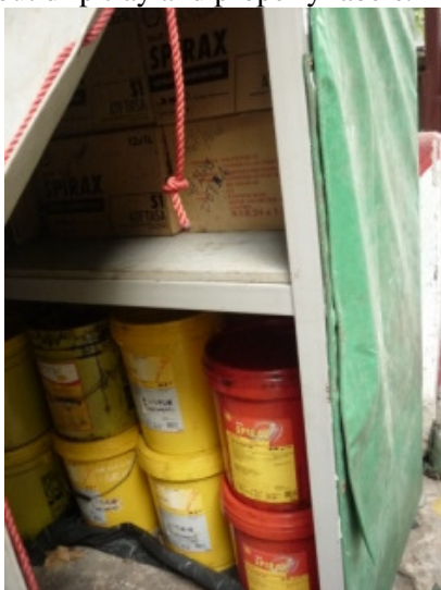
Photos 3 A chemical storage container was found without drip tray and properly labels.
