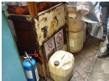
Photo 3 Oil drums were found without drip trays near noise enclosure.
