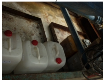
Photo 2 The drip tray had been provide to chemical under Aqua.Sed
