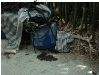
Photo 1 Oil stains were found on the floor near the chemical storage.
