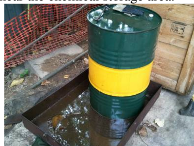
Photo 2 Accumulated water was found in the drip tray near the chemical storage area.
