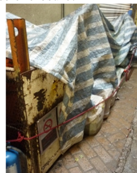
Photo 2 Oil drums were found without drip trays near noise enclosure.
