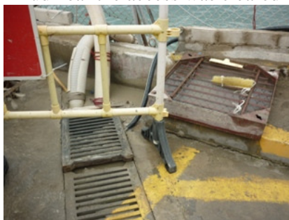
Photo 5 Mud near the access was cleared
