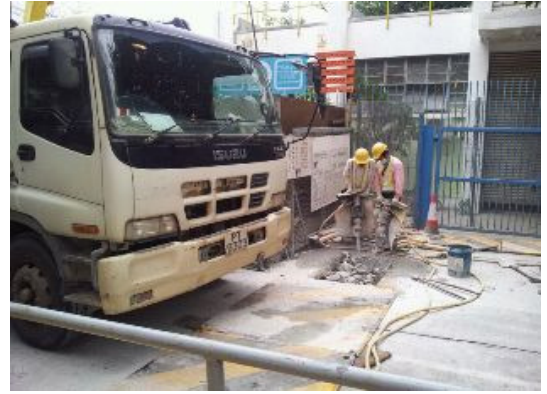
Photos 1 and 2 Rock breaking with using hand held breaker of other contractor
