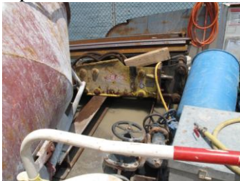
Photo 1 Accumulated water was found at the corner near the stockpiles since last inspection
