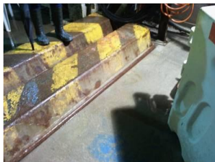
Photo 5 Water accumulation was found near access inside the noise enclosure
