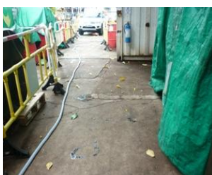
Photo 5 Water accumulation was found near access inside the noise enclosure
