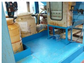
Photo 2 The chemicals near the Aqua Sep have been removed.
