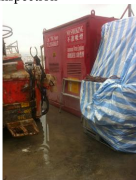
Photo 1 Accumulated water was found at the corner near the danger goods storage since last inspection
