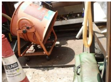
Photo 3 The accumulation waste was cleared
