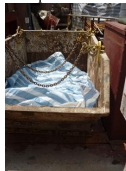
Photo 2 Water accumulation was found in skip on the noise platform
