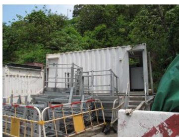
Photo 9 The sanitation level of the toilet was found poor
