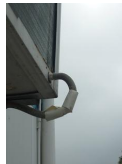
Photo 6 The contractor was using tape to temporary fix the pipe of air conditioner in PTW
