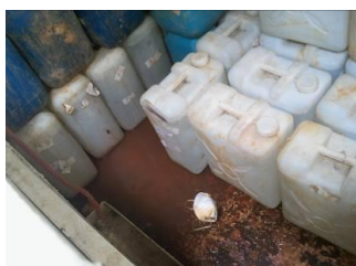
Photo 3 Some water accumulation was found in drip tray near the noise enclosure
