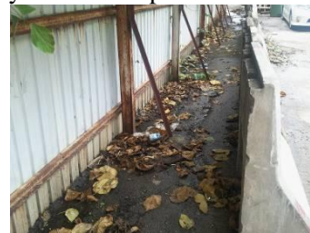
Photo 8 The trashes within 1.5m from the site boundary of workshop were cleared.
