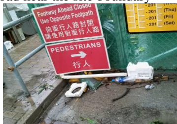
Photo 1 The trashes were found on the public access road near the site boundary
