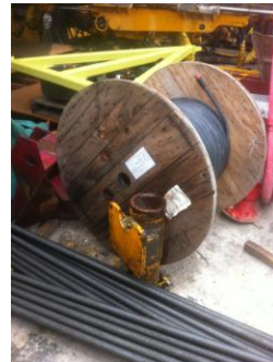
Photo 2 The contractor was reminded to clear stagnant water inside machineries.
