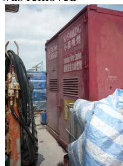
Photo 2 Accumulated water near danger goods storage was removed
