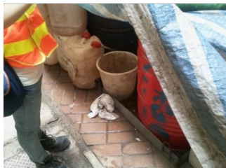
Photo 1 Chemical without drip tray were found on the access near the noise enclosure
