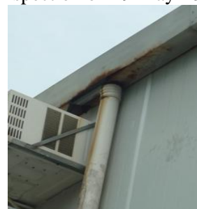
Photo 4 The dilapidation roof of site office was found to avoid the water leakage in PTW since inspection on 29 May 2012
