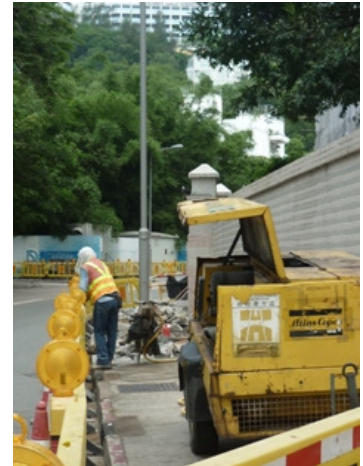
Photos 1 - 3 Road surface breaking with using hand held breaker of other contractor
