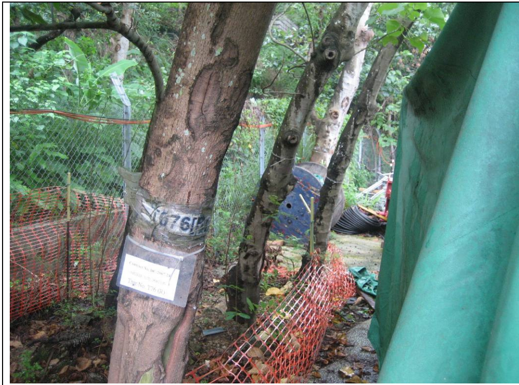
Aberdeen site --- Photo 9 Tree protect zone for the retained tree T076(R) and T077(R) was damaged.
