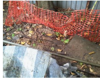
Photo 6 Water accumulation in the drip tray for containing oil droplet was found in the fuel storage area.
