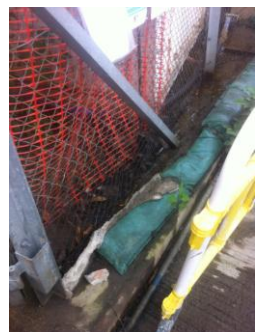
Photo 5 Stagnant water was found in the drip tray near the noise enclosure.
