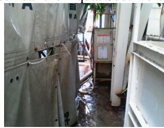
Photo 2 The stains on the noise enclosure surface and the wastes near the Aqua. Sed. were removed
