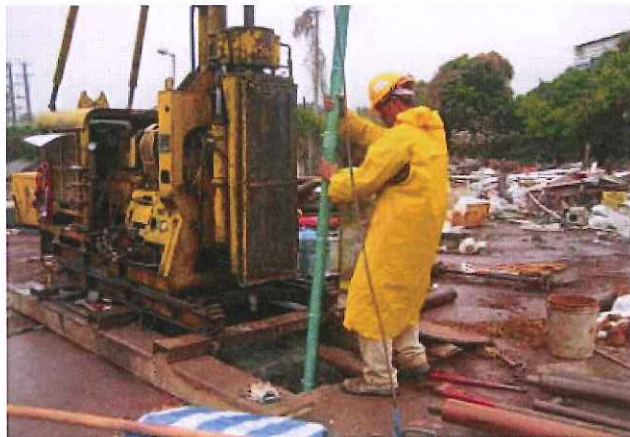
Photo 15 - Site G Temporary Groundwater Well Installation at G-06
