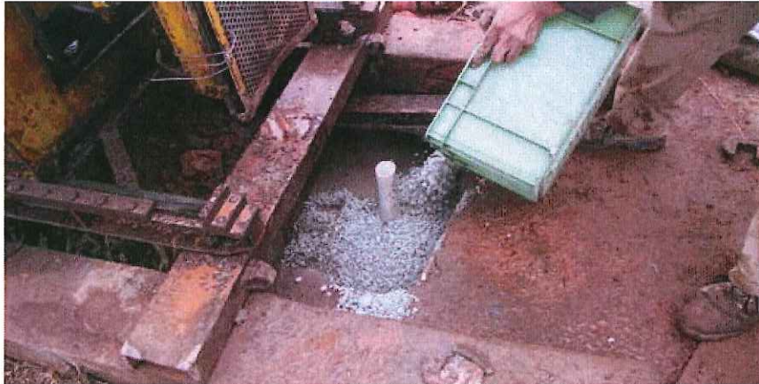
Photo 16 - Site G Temporary Groundwater Well Installation at G-05
