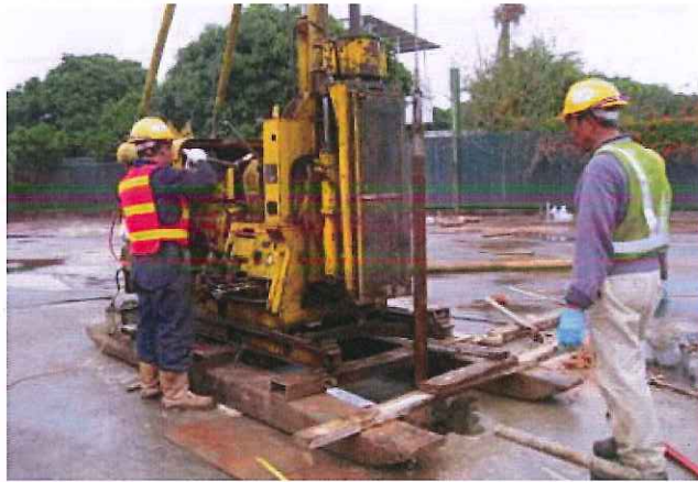
Photo 2 - Site F Drilling at F-05
