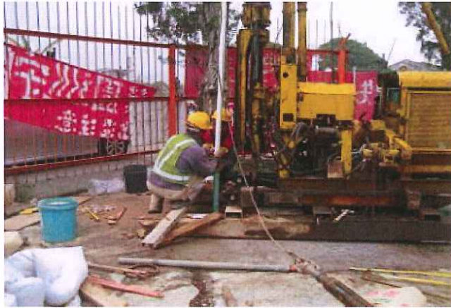
Photo 7 - Site F Temporary Groundwater Well Installation at F-06
