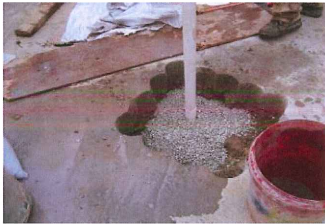
Photo 8 - Site F Temporary Groundwater Well Installation at F-07
