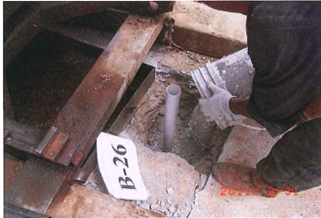
Photo 28 - Site B2 Temporary Groundwater Well Installation at B-26
