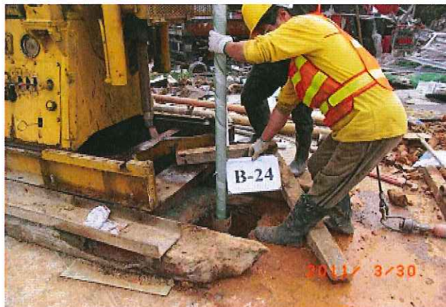
Photo 27 - Site B2 Temporary Groundwater Well Installation at B-24
