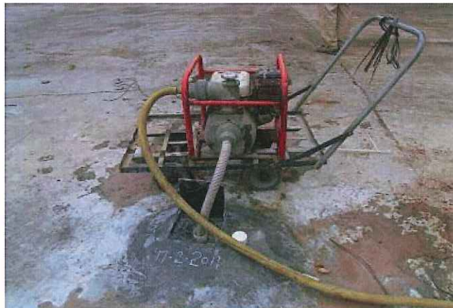
Photo 9 - Site F Purging at F-07
