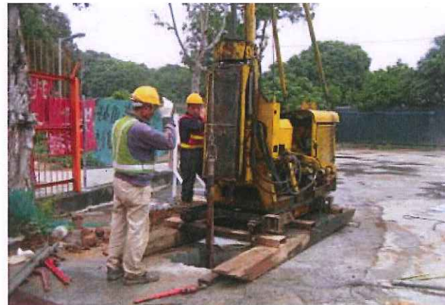
Photo 3 - Site F Drilling at F-06
